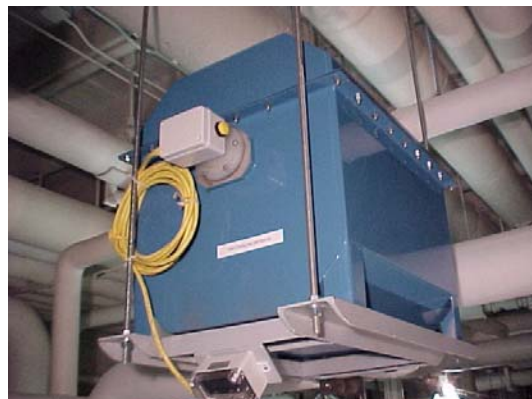
Pictured below is a new Stainless Steel "G" size condensate meter with a remote electronic counter
